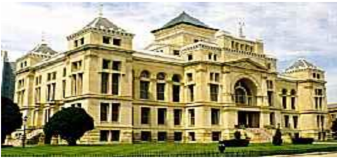
The Old Sedgwick County Courthouse
